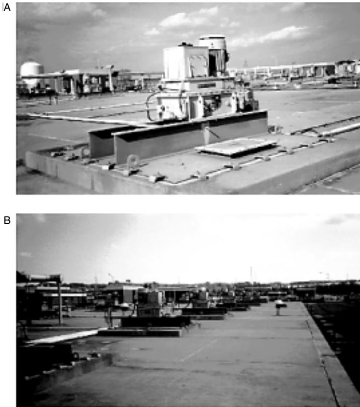
**FIGURE 1.2** (A) New surface aeration system for MCUA plant showing (B) compact surface aeration drives, (C) with elimination of most overhead piping, and (D) elimination of most equipment from compressor room. (Photos courtesy of Middlesex County Utilities Authority, Sayreville, New Jersey.)
