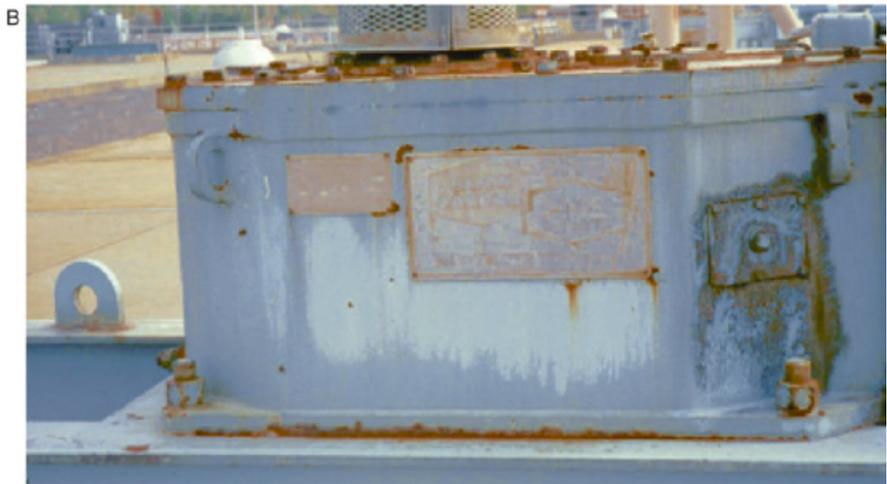
**COLOR FIGURE 1.1** Original submerged turbine system for MCUA plant showing (A) aeration tank turbine drives, (B) gear reducer.
